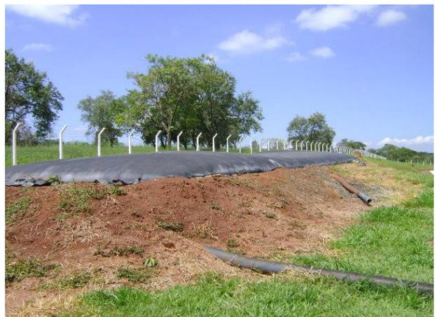
FOTO 4.10 – LODO DA LIMPEZA DA LAGOA ANAERÓBIA EM PROCESSO DE SECAGEM
